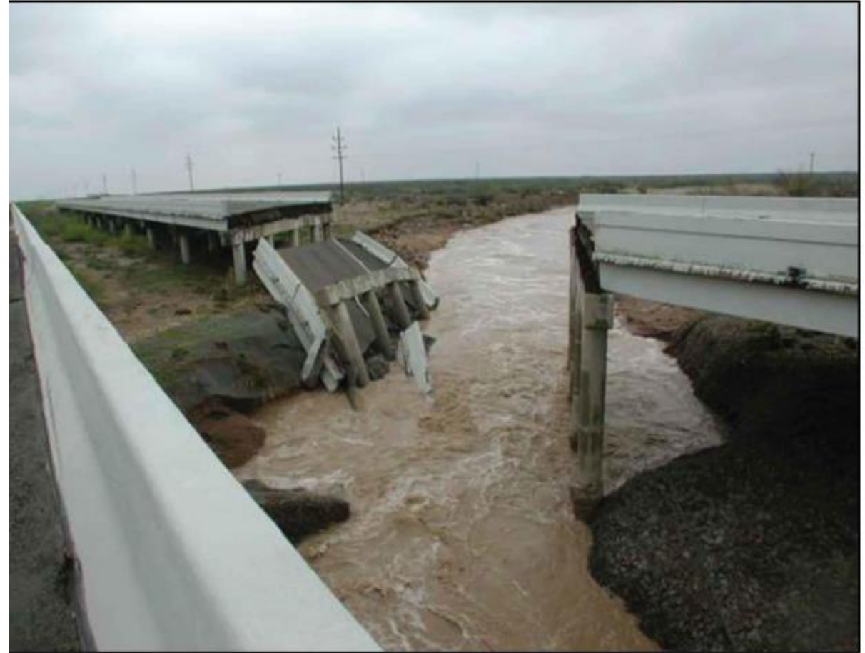
April 2004 flood caused this I-20 bridge over Salt Draw to collapse, located between Toyah and Pecos. Source: DAA and NWS; https://www.weather.gov/maf/2004_04_02_SevereWeather
