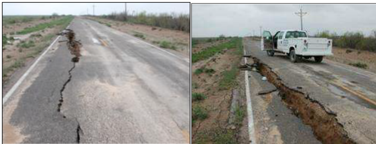
Sinkholes formed along this County Road southwest of Pecos, Texas during the April 2004 storm event. Source: NOAA and NWS; https://www.weather.gov/maf/2004_04_02_SevereWeather
